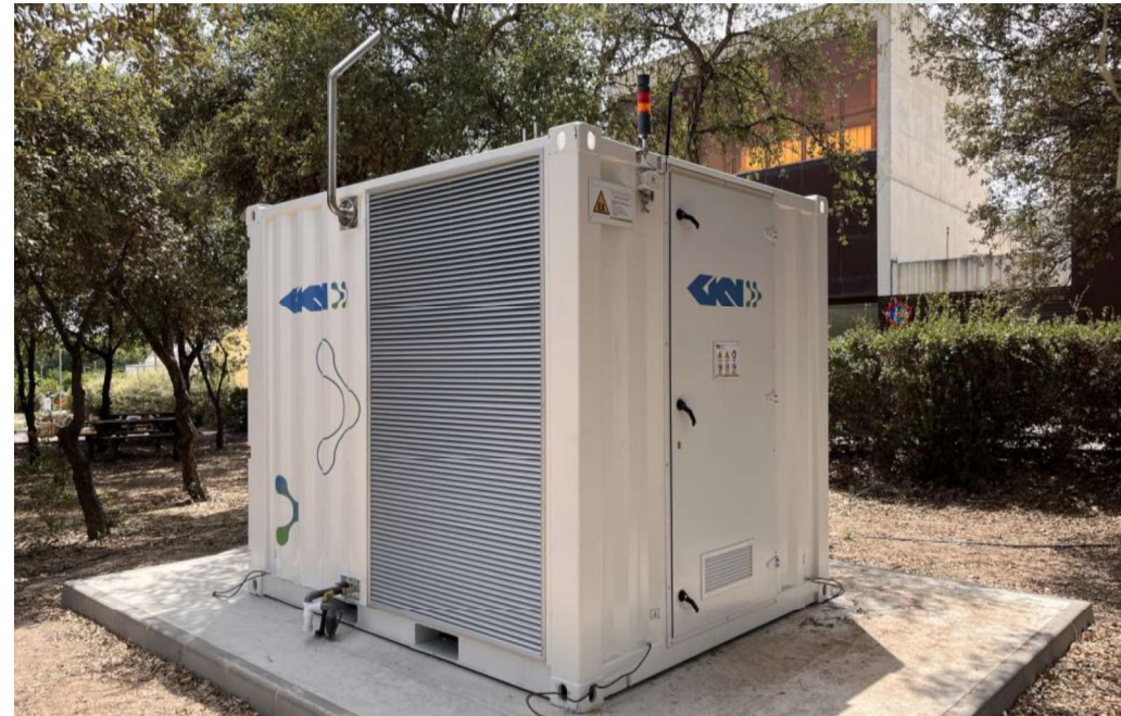
Plug & Play Power-2-Power System with Electrolyzer, Storage & Fuel Cell
